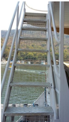
Stairs to top deck
